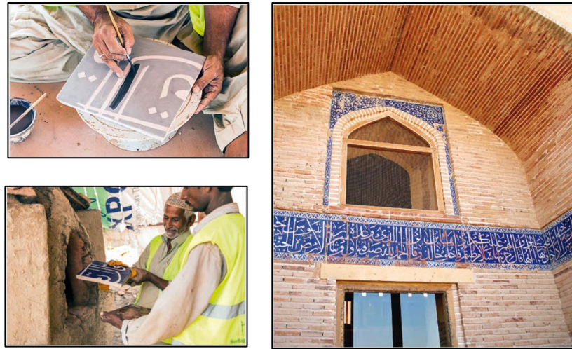
Figure 10. 17. Production of calligraphy glazed tiles for Sultan Ibrahim Mausoleum (left) and Sultan Ibrahim Mausoleum in Makli (right) (Resource: UNESCO/Heritage Foundation, cited in Han, 2018: 11)
